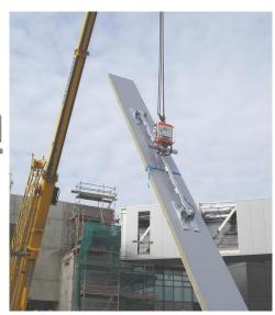
NOTE - As with all Clad Boy® vacuum panel lifters, the HD model has been proven to work effectively and safely with all industry standard panels, including mineral wool cored panels.
