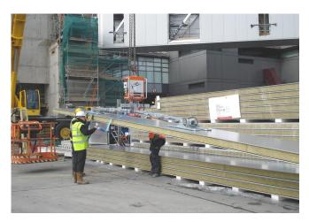
A more typical configuration utilises the double suction pads on traverse extension arms to provide increased panel support and in this form the unit can handle panels weighing up to 1320 lbs.
